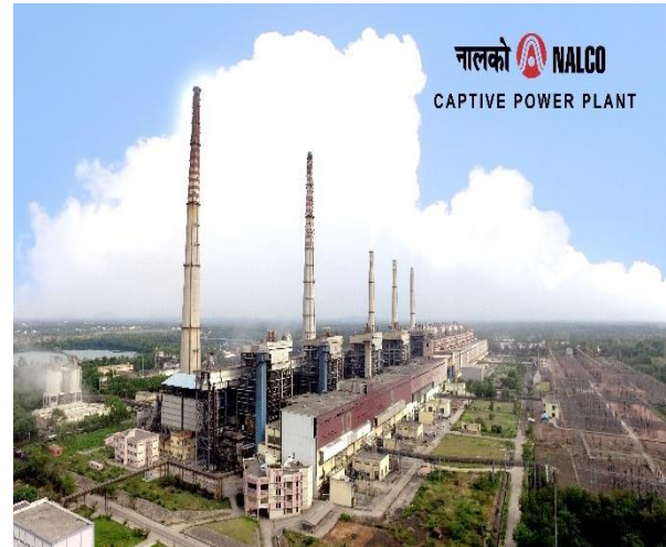
Photo -7.5 Captive Power Plant
