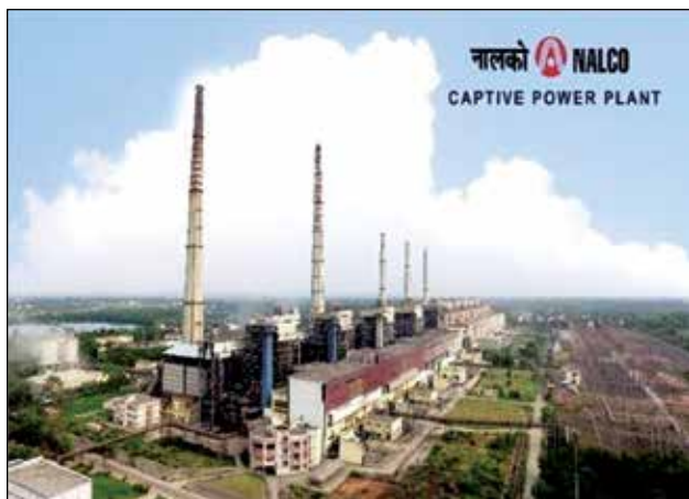
Photo-7.5 Captive Power Plant
