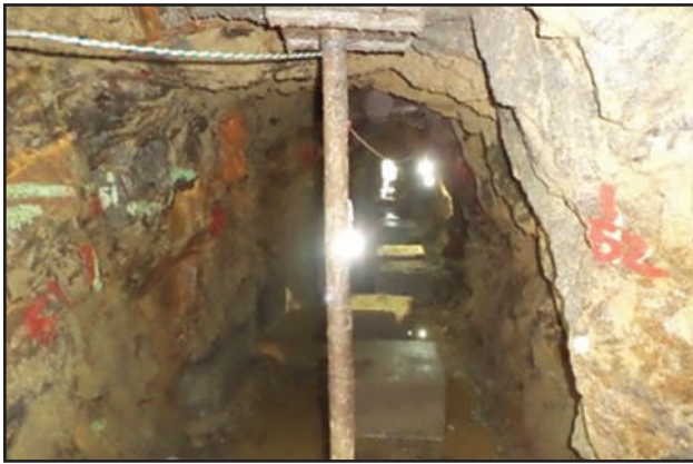
Photo 11.12: Exposure of granite gneiss in the right abutment exploratory drift [Loc. Mawblei HEP, Meghalaya].
