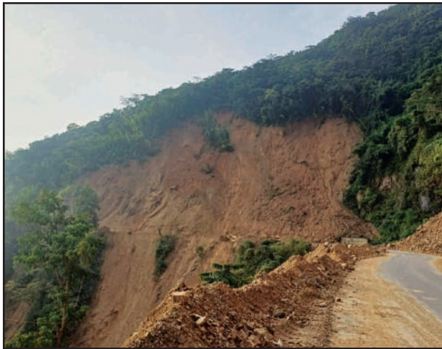
Photo 11.15: Debris slide along Thaizawl– Bualte road section posing risk to the road [Loc. Near Bualte, Lunglei District, Mizoram].
