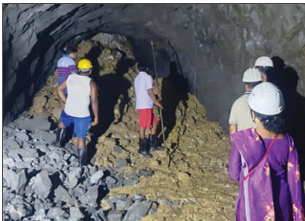
Plate 1 : 1 st Collapse from face-IV, ingress of debris flow on 7 th January 2023
