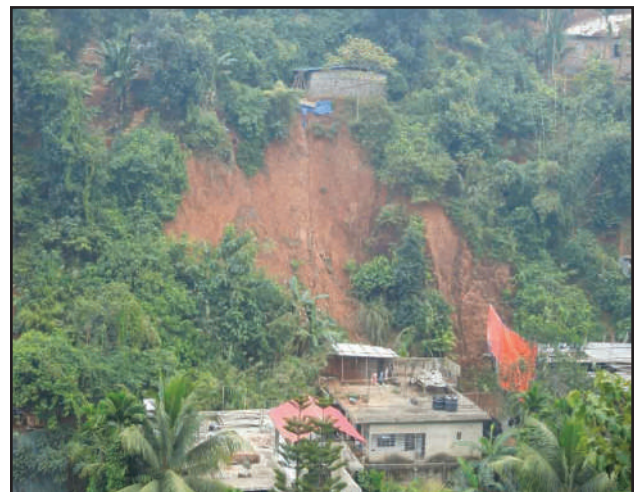
Photo 11.14: Shallow translational earth slide posing risk to settlement [Loc. Krishna Nagar, Kamrup (Metro), Assam].
