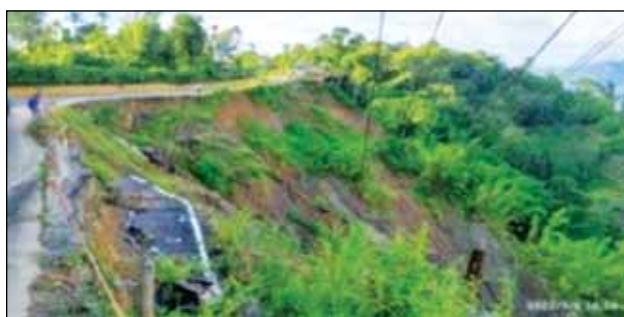
Photo 11.19: Field photograph showing sliding of slope forming material at the edges of road along Lumding-Badarpur section, Assam
