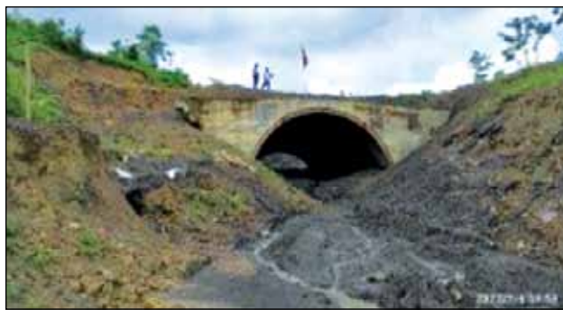
Photo 11.18: Field photograph of front portion of cut and cover tunnel section of Dimapur-Kohima new BG railway line, Nagaland.
