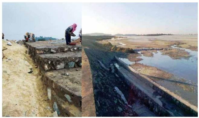
Photo 7.9 Heightening work of tailing dam retaining wall at MCP
