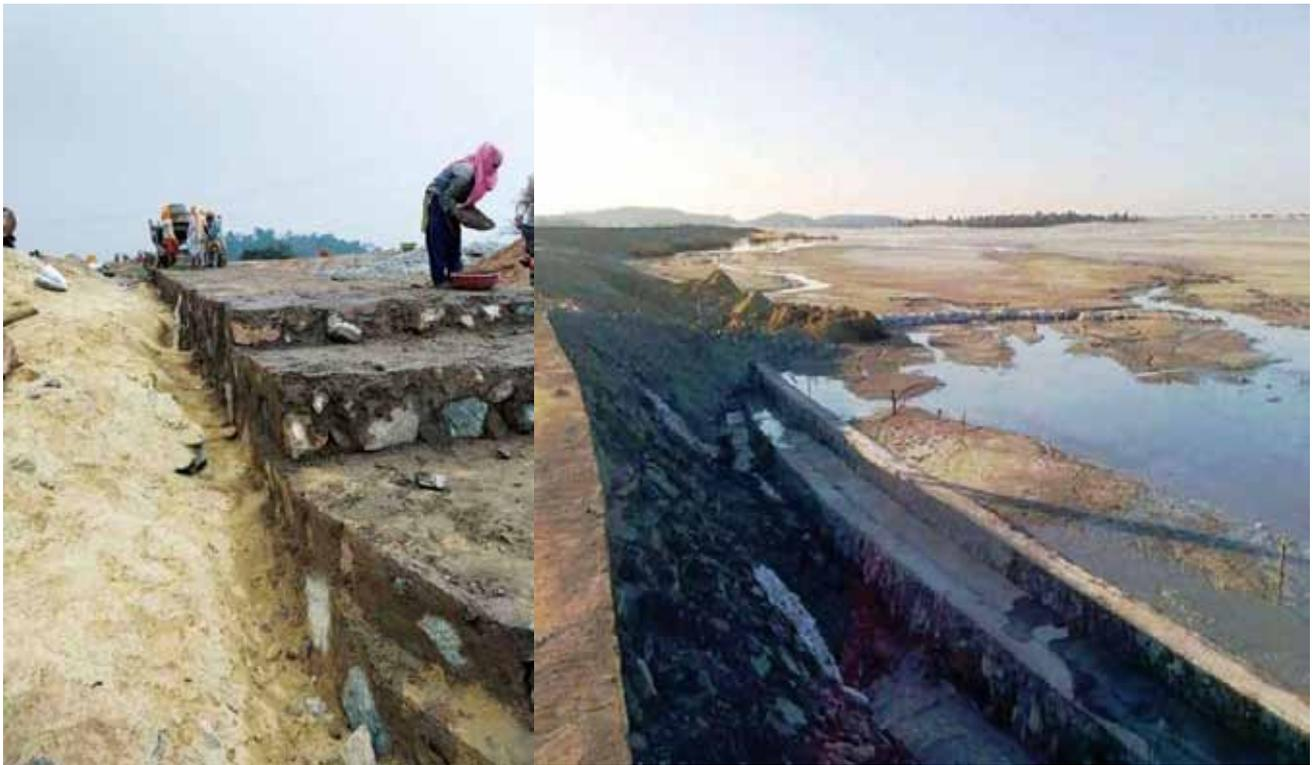
*Photo 7.9 Heightening work of tailing dam retaining wall at MCP*
