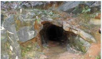
Photo.11.11 Exploratory drift on the right bank of Myntdu River (EL248.0m), Myntdu-Leshka stage-ll Hydroelectric Project
