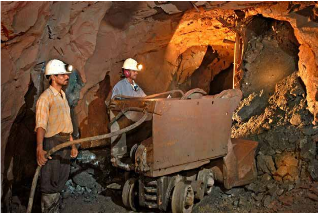
Run-of-Mine Mucking at Nuasahi underground Mines
