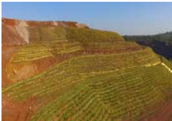
Stabilisation of Waste dump in an Iron Ore mine in District Keonjhar, Odisha
