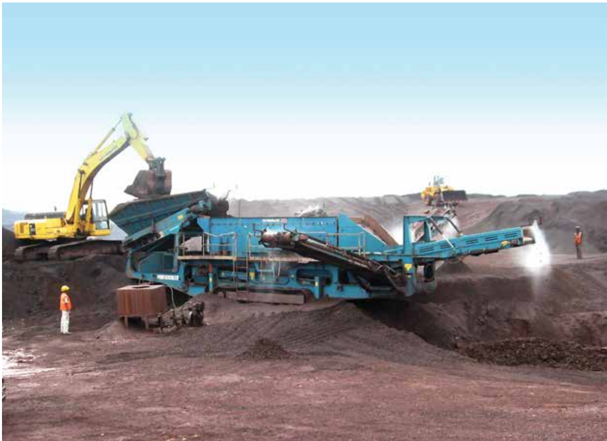
Mineral Conservation through in Pit Crushing
