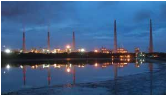
Captive Power Plant, Angul
