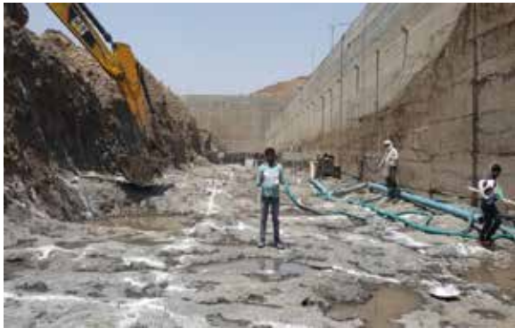
Foundation media at Apron portion of Mohanpura Multipurpose Project, Rajgarh, MP
