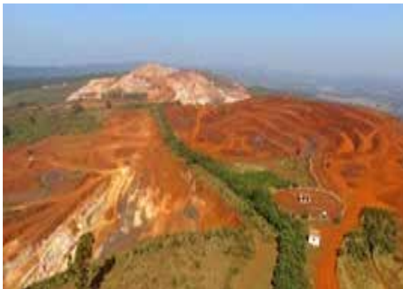
Safety Zone Plantation between lease boundaries of 3 iron ore mines in Odisha
