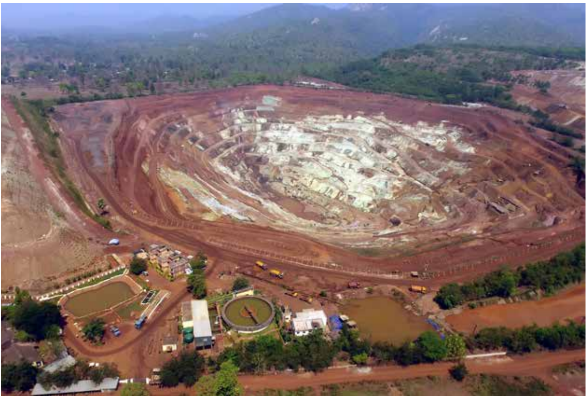
Aerial view of Chromite mine along with ETP
