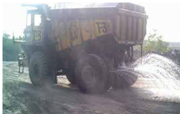
Water Sprinkling on Roads
