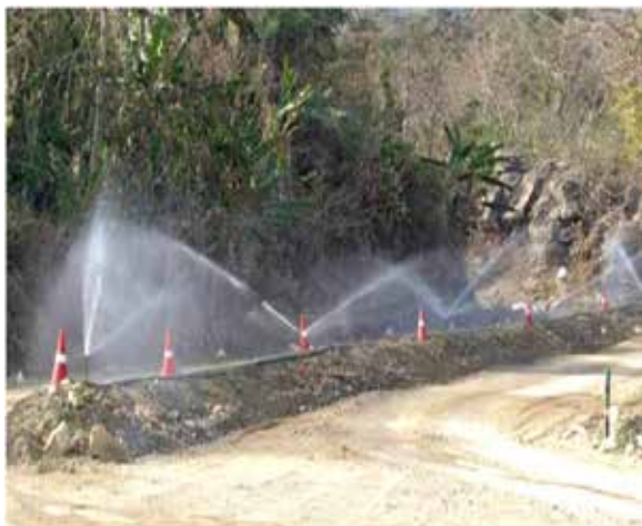
Water sprinkling on haul roads
