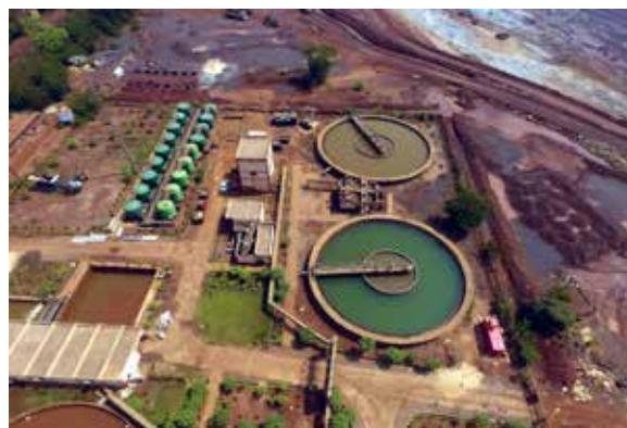
Effluent Treatment Plant in Chromite mine
