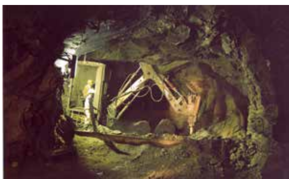
Underground mines of KCC
