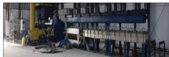
Stage-wise erection and commissioning of 14MN Extrusion press at JNARDDC, Nagpur
