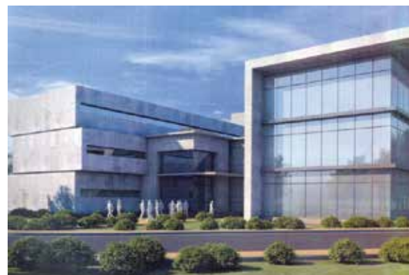
The new Laboratory Complex of MECL at Nagpur
