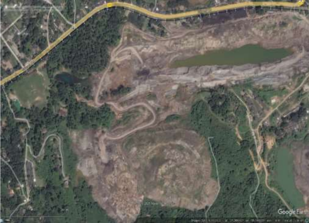
Ledo OCP during Operation
