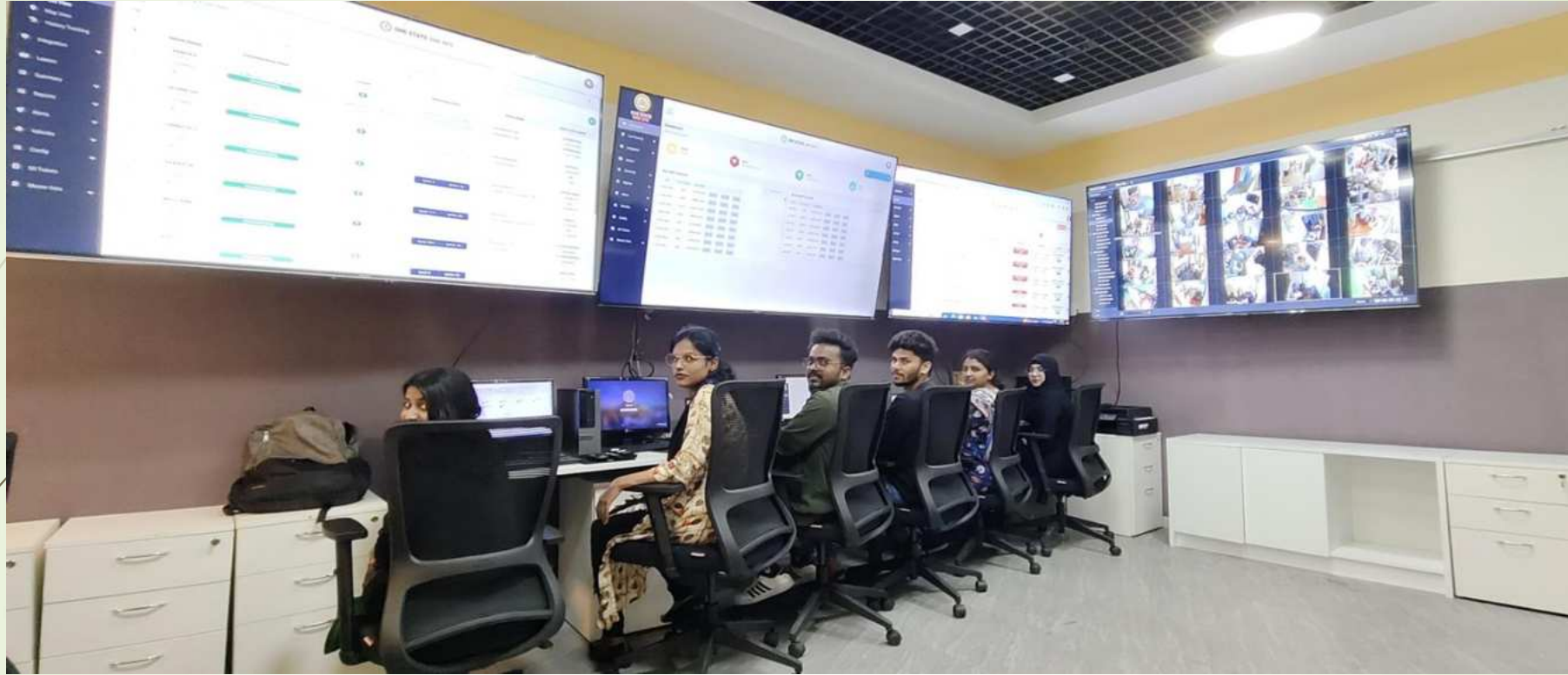
View of OSOG Control room
