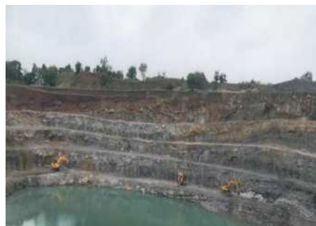
BENCHING PATTERN IN DOLOMITE MINES
