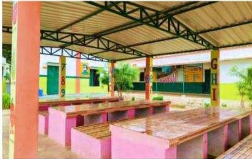
Infrastructure Development at Mahuari Kalan Primary School
