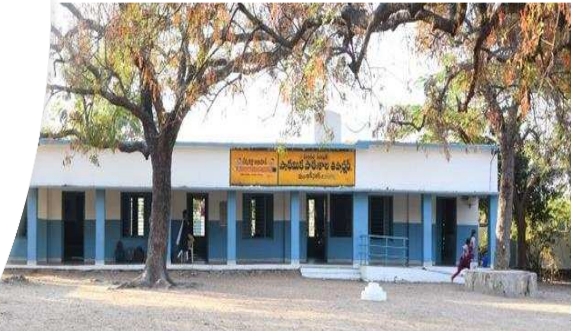
Painting and repairs in school buildings
