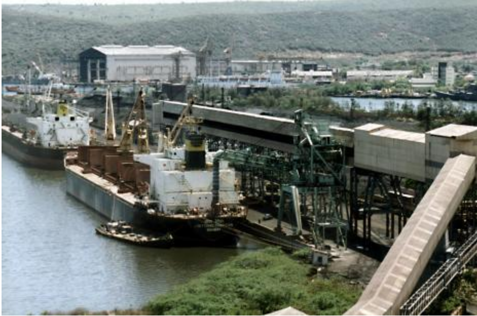
Figure 2 : Port Facilities, Vizag
