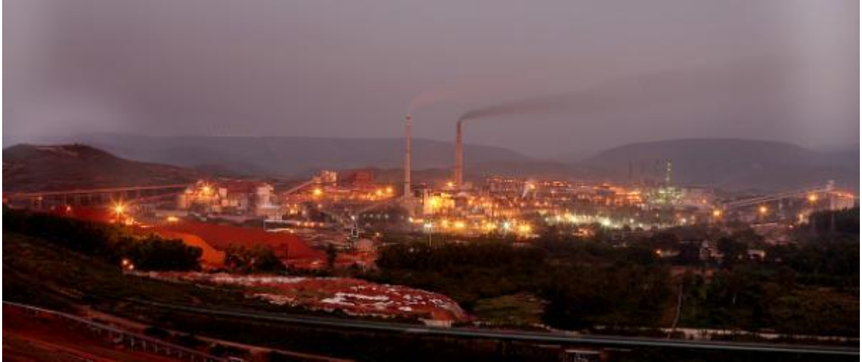
Figure 4 : Alumina Refinery, Damanjodi
