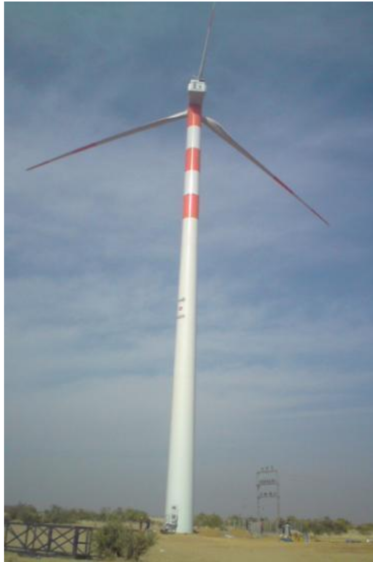
Figure 7 : Wind Power Plant, Jaisalmer
